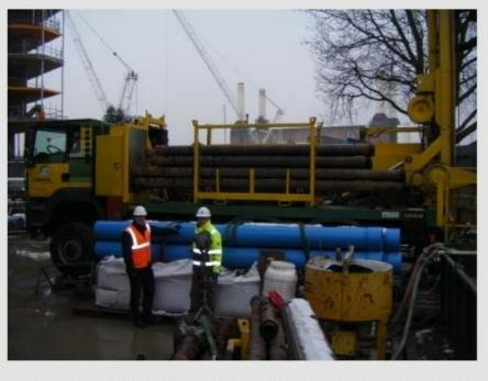
Boode's 330mm OD x 292mm, 19.5mm wall thickness (heavy wall) PVC casing deals with the grouting and onward drilling phase without issue. Approval under Regulation 31 of the Water Supply (Water Quality Regulations) means that, should the wells ever be required for potable water abstraction they are already compliant. The cylindrical perfection of Boode's PVC casings simplifies the drilling & installation process, one of
