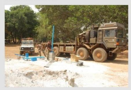
Installing each pump takes around six days and there are eleven sites to cover. As each borehole is drilled the engineers will line the new well with Boode PVC Screen with a high quality quartz silica filter pack, Boode PVC Casing and install the robust, long life hand pumps.
